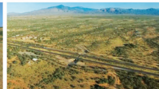
Full-interchange and underpass tunnel at the northwest corner
